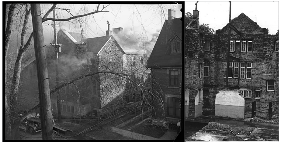
FIG. 5. SUNDAY SCHOOL HALL FIRE, EXTERIOR AND GUTTED INTERIOR, DOMINION-CHALMERS UNITED CHURCH. | PHOTOGRAPHER UNKNOWN. COURTESY OF DOMINION-CHALMERS UNITED CHURCH ARCHIVES.
