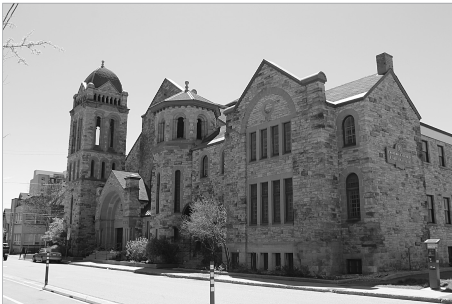
FIG. 3. DOMINION-CHALMERS UNITED CHURCH, 355 COOPER STREET, OTTAWA, MAIN FAÇADE, LOOKING SOUTH ON O'CONNOR STREET. | NATALIE ANDERSON RATHWELL, 2017.
