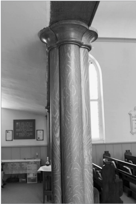
FIG. 31. GALLERY PIERS, HOLLAND LANDING. | ALANA DUGGAN.
