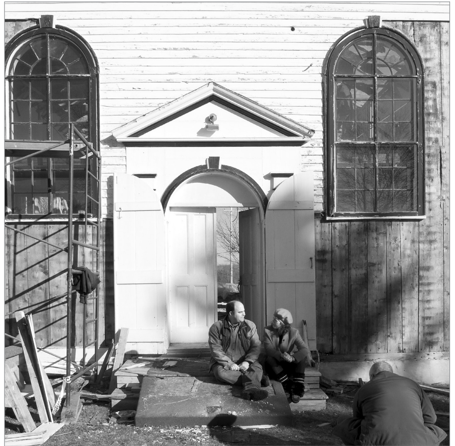
FIG. 10. RYAN SCRANTON AND COLLEEN JONES WITH A CBC CAMERA OPERATOR AT ALL SAINTS, GRANVILLE CENTRE, DURING THE DEMOLITION IN 2009. | PETER COFFMAN.
