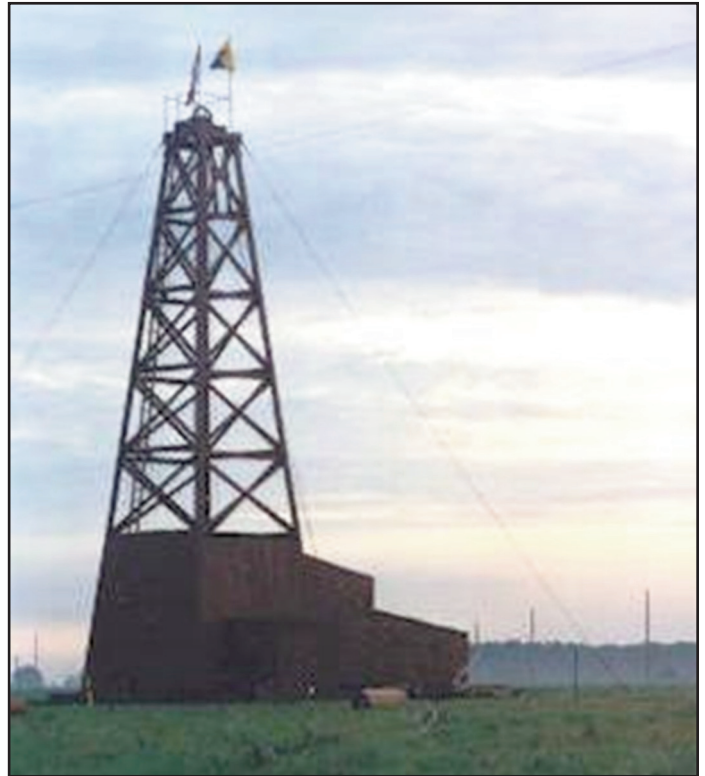
Figure 3. Canadian Drilling System rig rebuilt in 1996.
