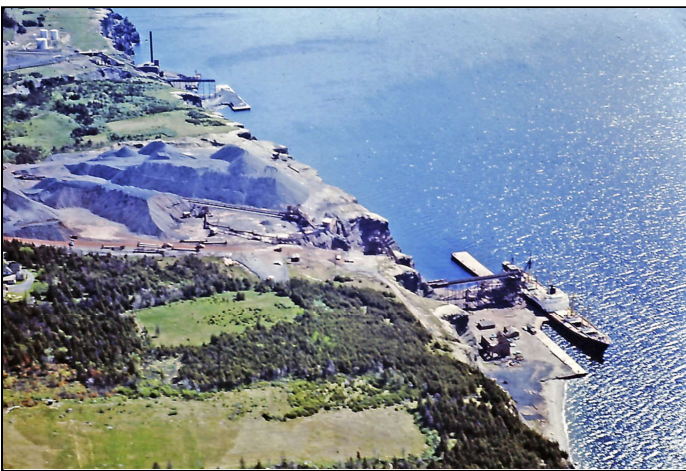
Figure 19. Abandoned Dominion pier (background), stockpile for ore storage (centre), and active Scotia pier (foreground). Source: Memorial University of Newfoundland–Digital Archives Initiative.
