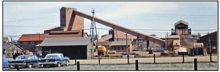
Figure 20. No. 3 mine deck head and float-sink mill and infrastructure added during mine expansion and modernization in the late 1950s. Source: Memorial University of Newfoundland–Digital Archives Initiative.
