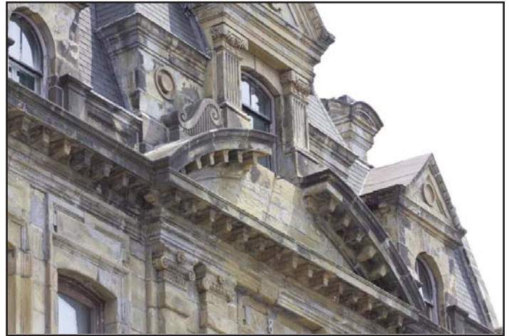
Figure 5. Building stones in Uptown Saint John connect the community to its history of a dimension stone industry.
