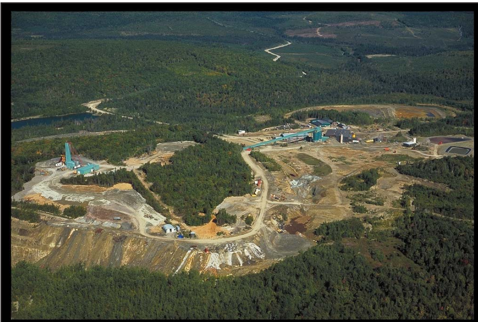
Figure 3. Aerial view of the Caribou Mine (circa 1997).
