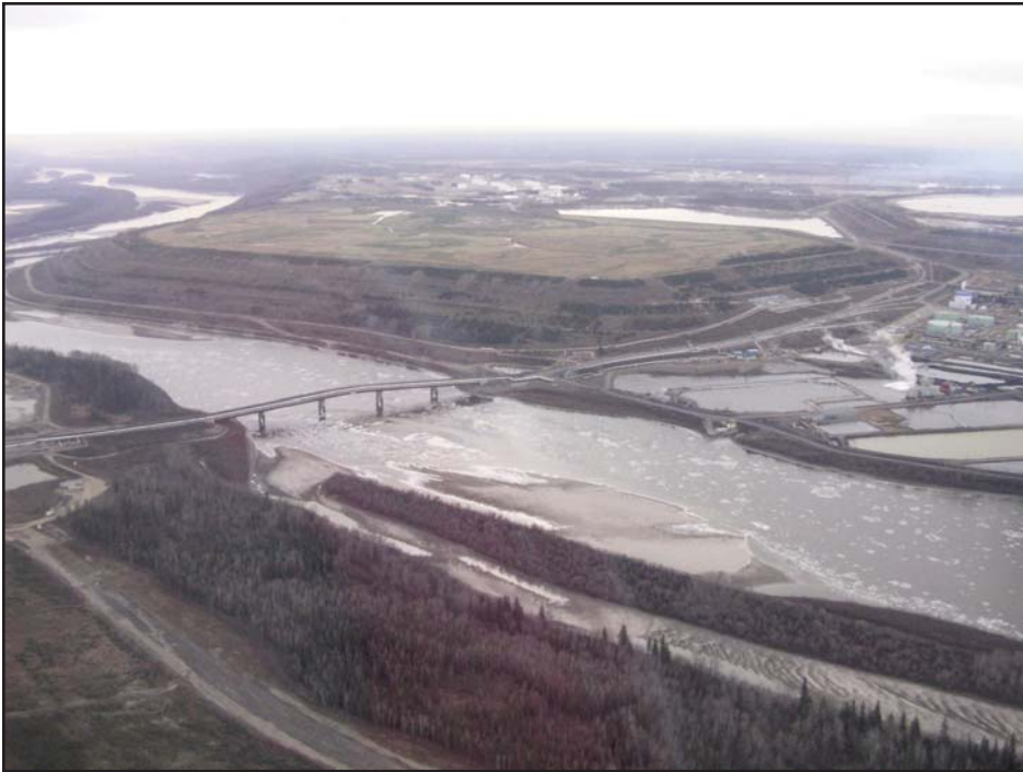
Figure 15. View west across the Athabasca River showing the Suncor Voyager Plant and Pond #1, in November 2010, restored to a dry state with a grass cover (photo by author during inspection visit as part of the work of the federal Oil Sands Advisory Panel).
