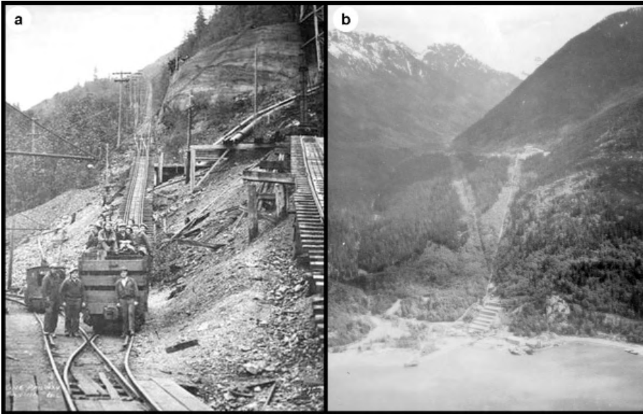
Figure 15. a. Rail car at bottom of the incline, loaded with freight and passengers, circa 1920. BMM Archives 996.11.2. b. View looking East up Britannia Creek showing Britannia Beach, Mill No. 3, the incline and Incline Camp at the 2700L, Goat Ridge (with snow) north of Britannia Creek and Britannia Mountain south of the creek. The 5.6 km-long electric railway went from the top of the incline to the Townsite on Britannia Creek 165 m higher. The Jane Mine was beyond the visible side of Britannia Mountain, 4.2 km from the mill on a straight line from Britannia Beach that passes just to the right of the Incline Camp. 1927 City of Vancouver Archives, Item Add. MSS. 75, Vol. 34.
