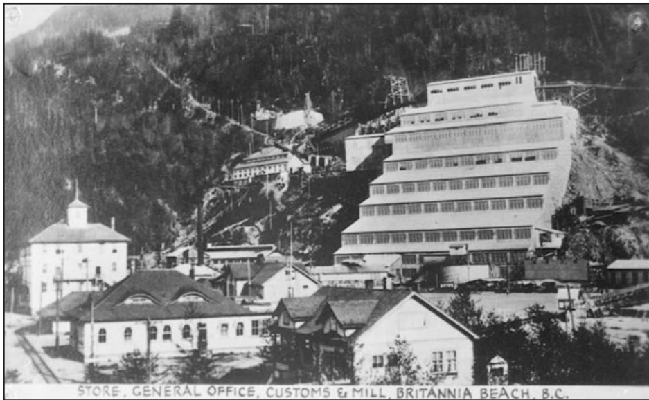
Figure 17. Mill No. 3; the co-op store, with the cupola, is on the left; incline cut is seen at top left of mill; circa 1925. BMM Archives 984.33.33.
