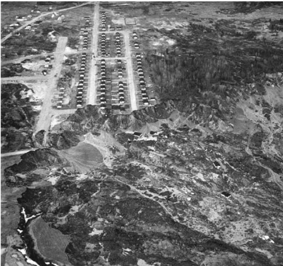
Figure 9. ‘Quick clay’ failure at Saint-Jean-Vianney, Québec, 1971. Photo by S.G. Evans.
