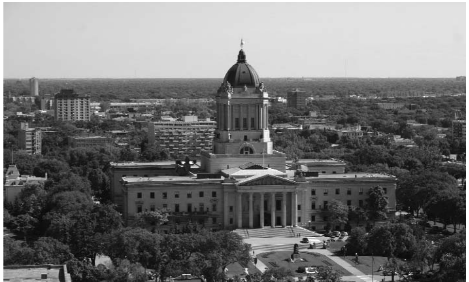
Figure 4. The Manitoba Legislative Building viewed from the north in spring 2005. Visitors are greeted at the front entrance by six ionic columns capped with a pediment symbolizing Canada. A sculpture of Queen Victoria, seen on the front lawn of the building, is one of many sculptures on the grounds. The refurbished Golden Boy atop the building symbolizes Manitoba's eternal youth and progress. Government House, the residence of the Lieutenant-Governor of Manitoba, is located on the left side of the photograph.
