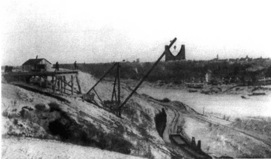
Figure 6 Siding from the Edmonton, Yukon and Pacific branch of the Canadian Northern Railway for the delivery of steel and stone for the Alberta Legislature. A five ton stiffleg derrick handed materials from the cars to a trestle and light railway on the top of the hill. To the southeast across the North Saskatchewan River the skyline of the town of Strathcona can be seen (Provincial Archives of Alberta, A 11017).
