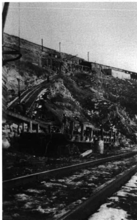
Figure 7 The Glenbow Quarry, 25 km west of Calgary on a siding from the Canadian Pacific Railway in the Bow River valley. Stone, quarried towards the crest of the valley was cut and trimmed in the shops below before being carried by the inclined tramway to loading facilities on the railway spur (Glenbow Archives, NA1025-1).
