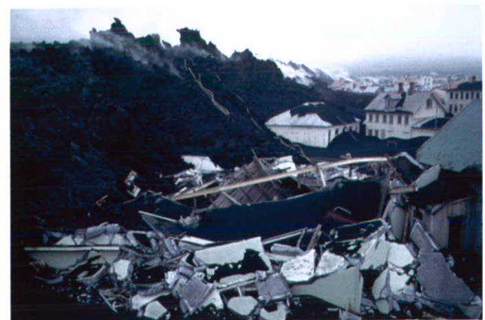
Figure 5 The lava advance into the town destroyed several hundred buildings including reinforced concrete structures in the harbour area. Cooling hoses can be seen on the lava front in the centre of the photograph.
