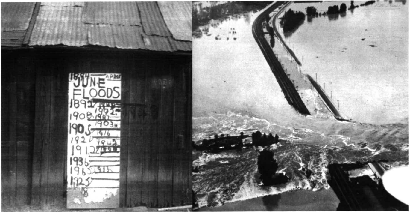
Figure 4a Telling the story with pictures (from Geoscape Vancouver ; Turner et al., 1996a). (left) Levels reached by Fraser River floods on a barn in the Fraser Valley since 1894 (British Columbia Ministry of Environment). (right) Dyke breach in the Fraser Valley during the Fraser River flood of June 1948 (Vancouver Sun/Dave Buchar).
