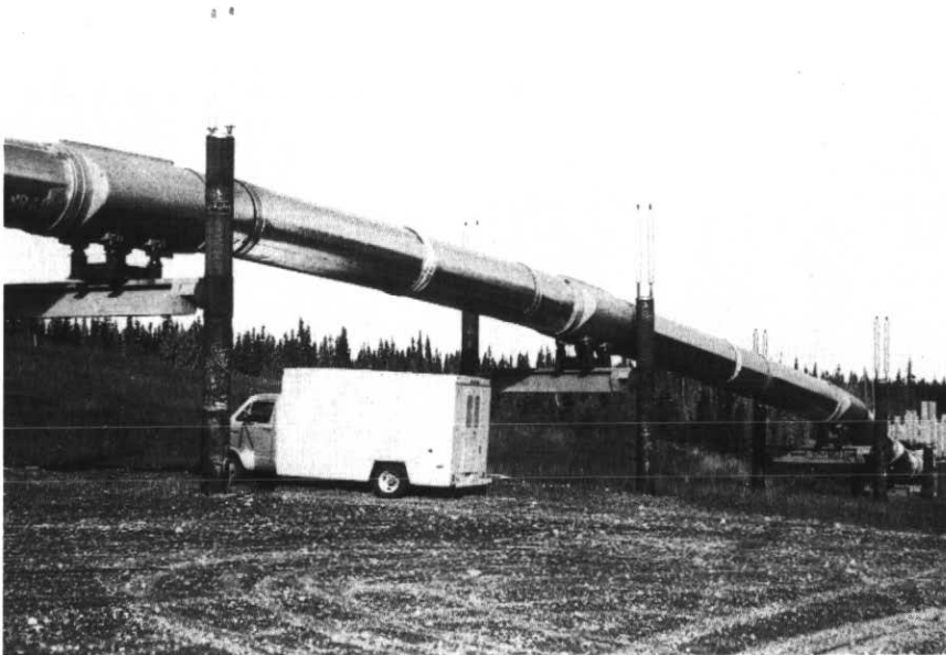
Figure 10 Trans-Alaska oil pipeline using vertical support members (VSMs) with cooling devices (fins) designed to prevent heat transfer to ice-rich, thaw-sensitive permafrost.
