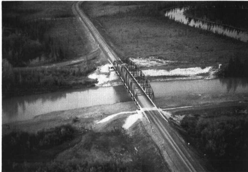
Figure 8 The Eagle River bridge, Dempster Highway, Yukon. This is a single span structure with minimal pile support in the river.
