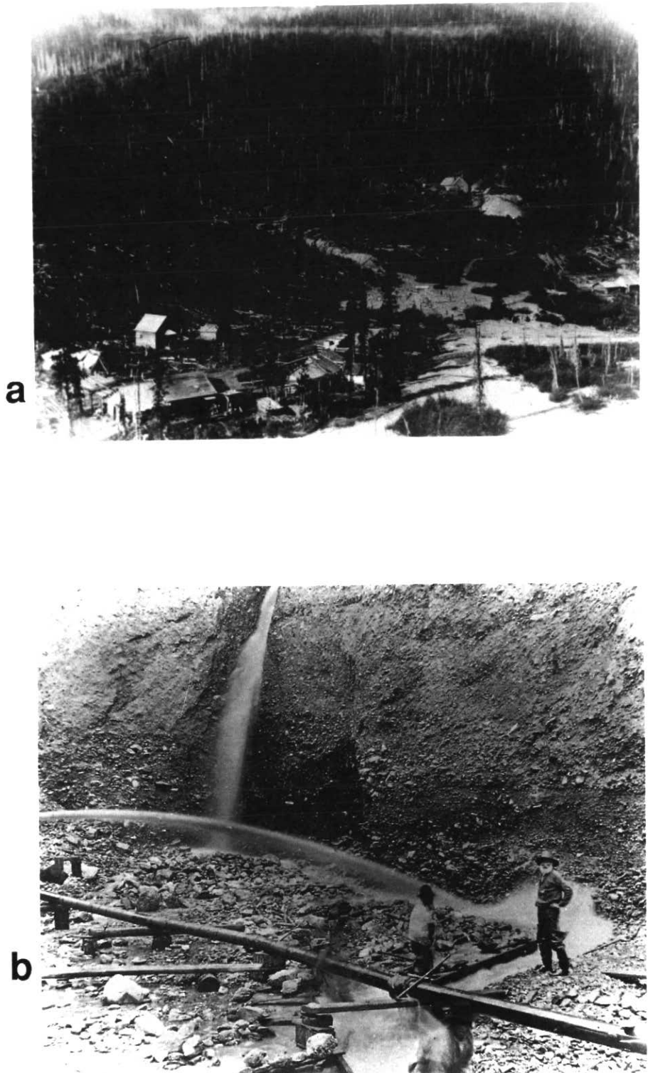
Figure 5 (a) (upper) Townsite at the base of Lowhee Creek just south of the present town of Wells, 1920s. (b) (lower) Hydraulic mining lodgement till and underlying gravels on the upper part of Lowhee Creek, 1930s.
