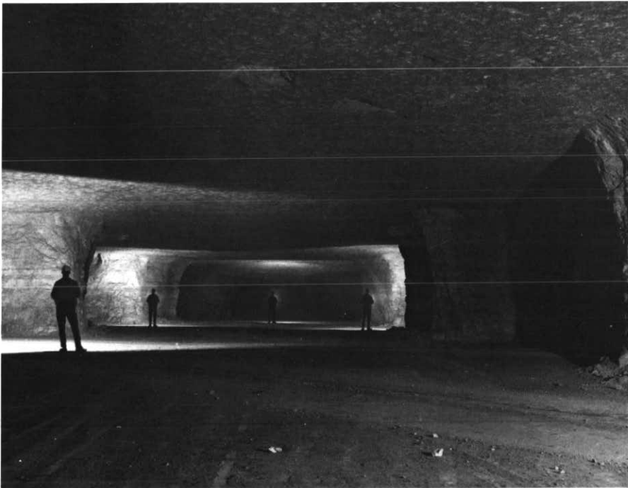
Figure 2. View inside one of the disused mined-out areas at Kansas City in the Bethany Falls limestone. This shows a level floor and competent rock roof; developments noted in
