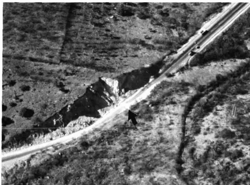
Figure 4 Road crossing of the fault, looking north. The far side has moved left, as confirmed by the offset in the white centerline of the road.
