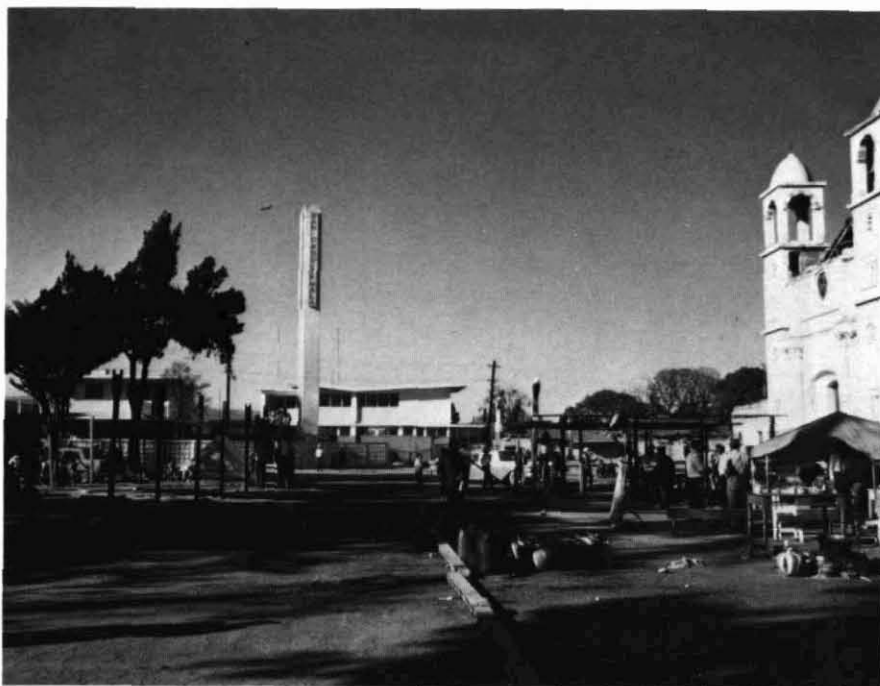
Figure 6 Chimaltenango: modern bank building and decorative brick wall remained standing.
