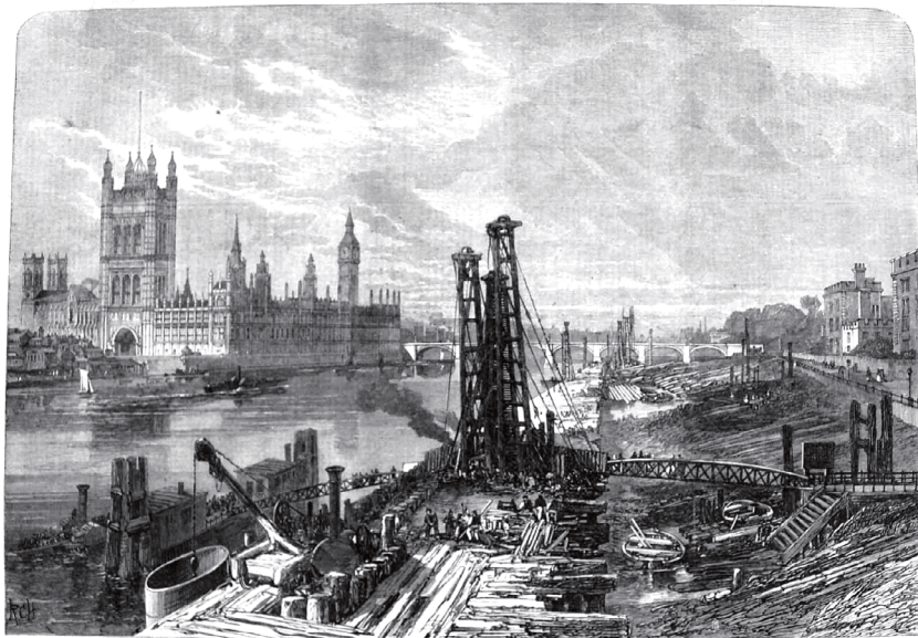
PROGRESS OF THE SOUTHERN APPROACH OF THE TRAMWAY AT LAMBETH — 100 POUNDING PAIR
