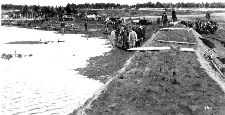
Figure Eight: Building a dyke at Long Island, Kings County, N.S. [PAC]
